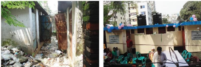
Pre & Post view of 13 Huts camp Toilet
